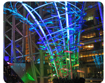
These metal atrium trees were designed in Cobalt and fabricated in China, using Cobalt CAD drawings and 3D models as a "production language" easily understood by non-English craftsmen.
